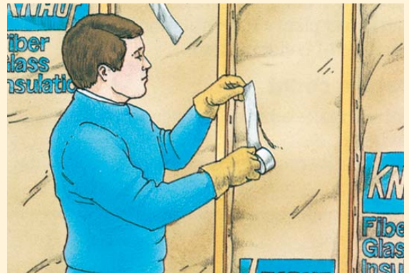
Patch any tears in vapor retarders.
