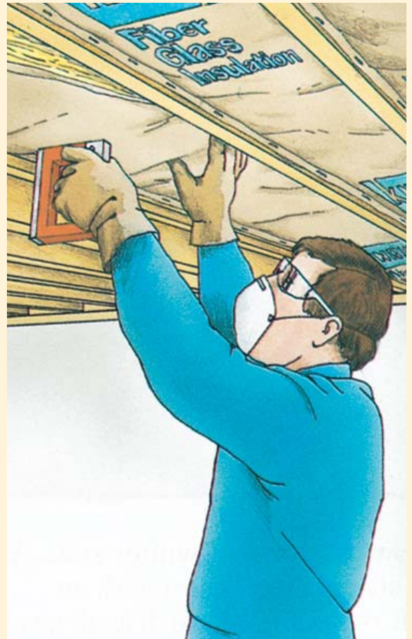
INSULATING CEILINGS: Staple the flanges of Knauf kraft-faced insulation to the inside of ceiling joists.
