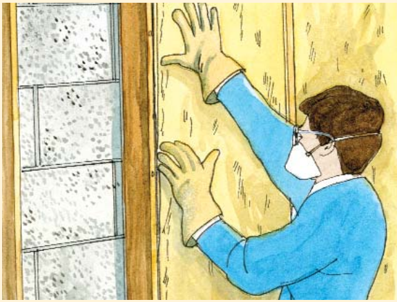
INSULATING BASEMENTS: Staple flanges every 4" to 6" along both sides of studs.
